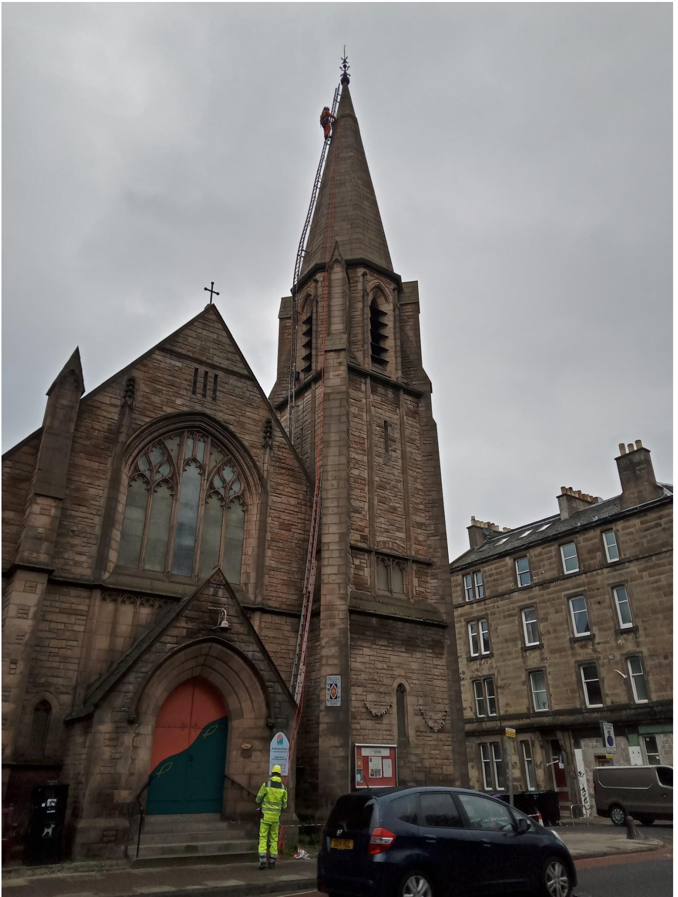
The work in progress to repair the spire and roof.
